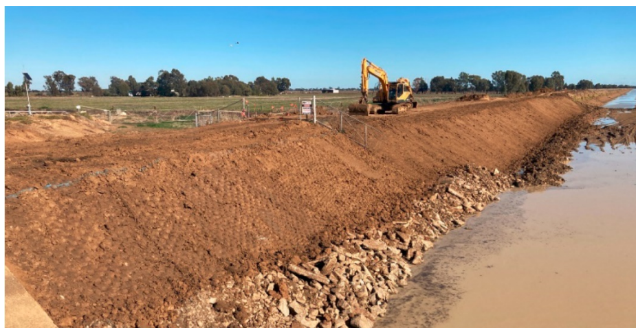
Bank reprofiling works on the Mulwala Canal repairing erosion
